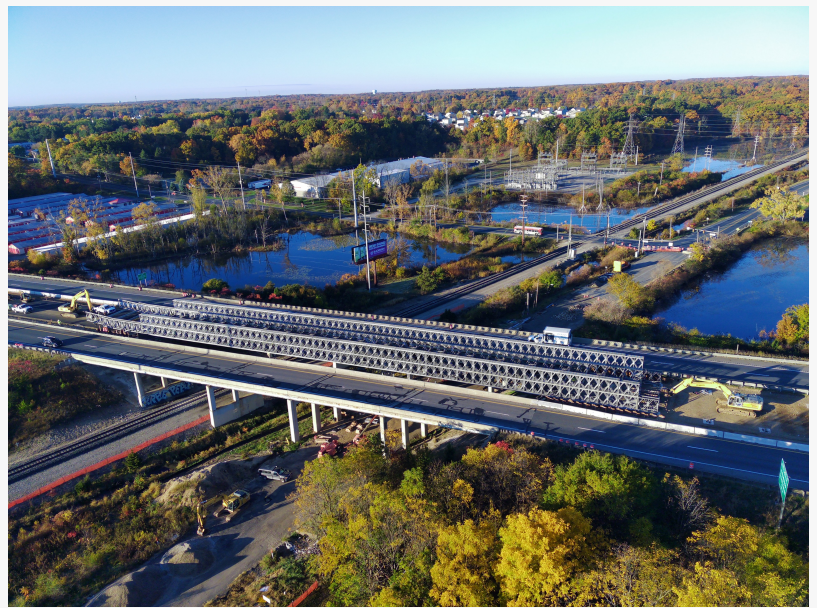
Acrow Bridge in service in Michigan
