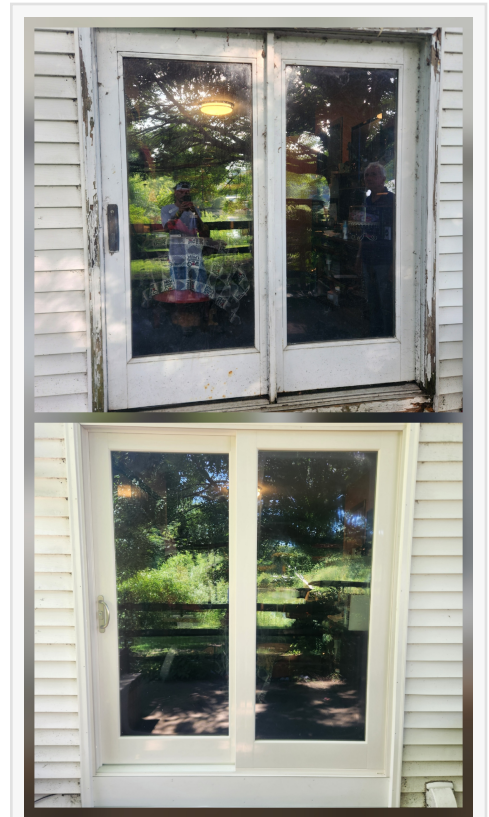
A before-and-after comparison of a recent energy-efficient window replacement completed by Hatfield's Seamless Gutters LLC.
