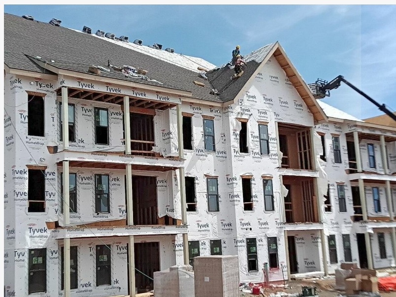
Roofers installing a Tamko Heritage Shingle in Weathered Wood on New Construction Project
