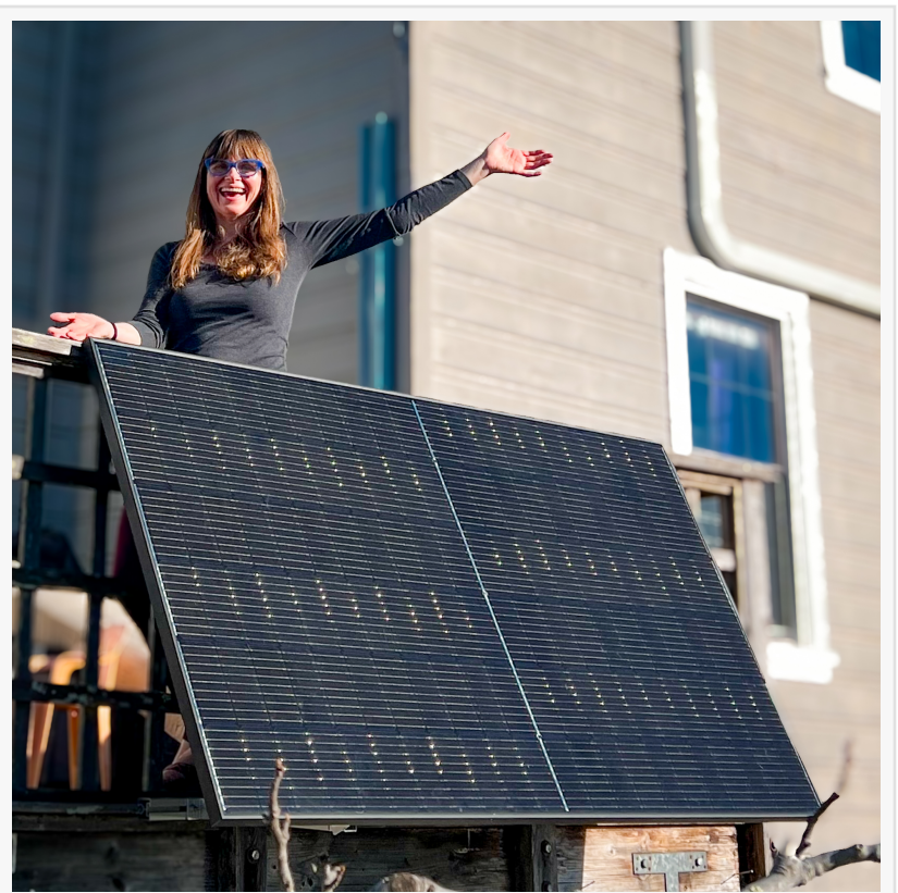
Plug-in solar panel installed on a balcony
