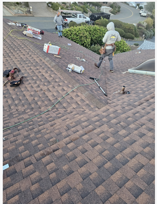
Roof City Inc installing new shingles. Quality roof replacement and repair services
