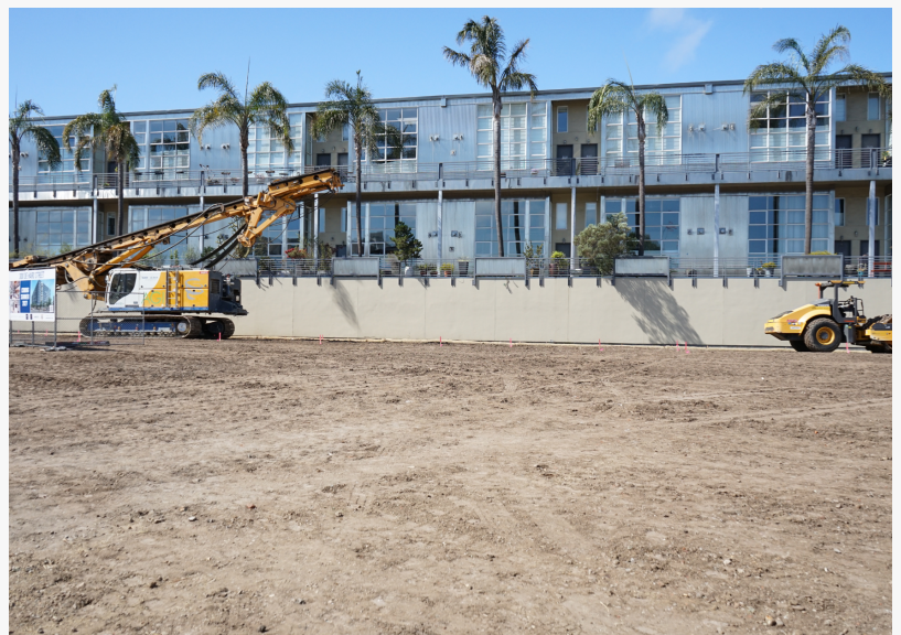
300 De Haro Street Construction
