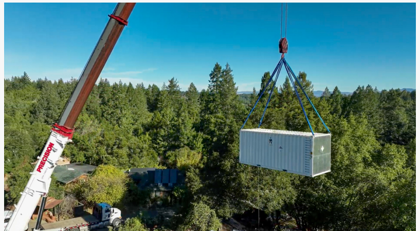
The battery storage system was lifted by a crane into position on the farm.
