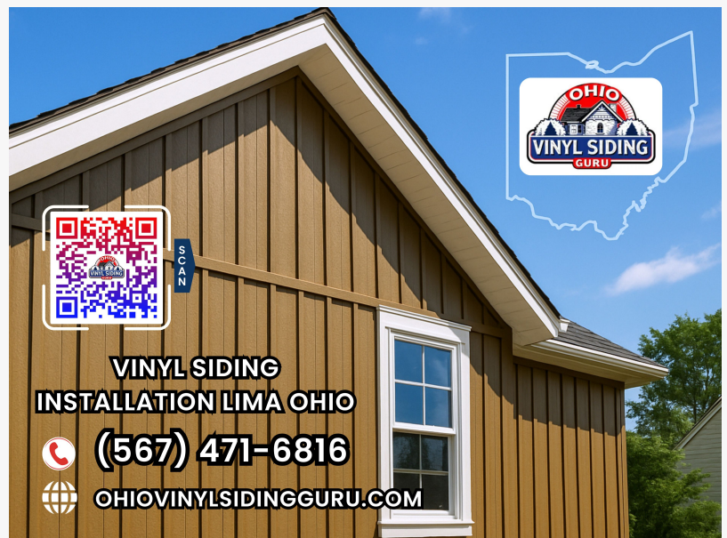
Vinyl Siding Installation in Lima Ohio
