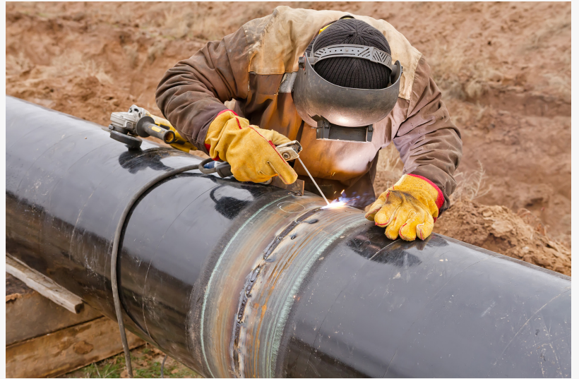
Welding Pipeline without Use of Additional Primers
