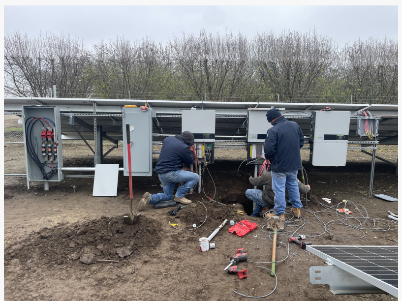
A1 Contractors installing a ground-mounted solar power system with inverters.
