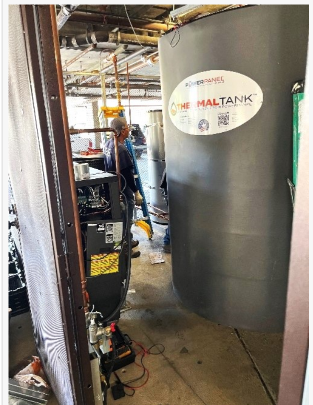
Thermal Tank installed on-site at the project. Its modular 'building block' design enabled the team to hand-carry it in and easily set it up in a tight space, in a fraction of the time a conventional tank would need
