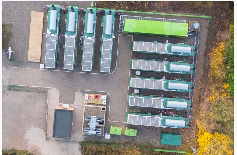
Terra Firma Energy's 9 Hydrogen ready Finning CAT sets at their 20MW flexible generation site in Wrexham, UK.
