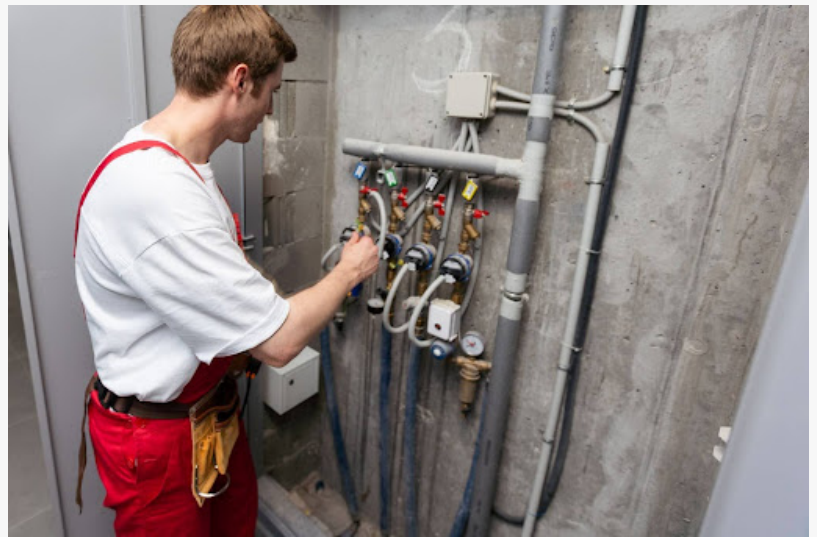
Plumber tightening a residential water meter connection using an adjustable wrench.
