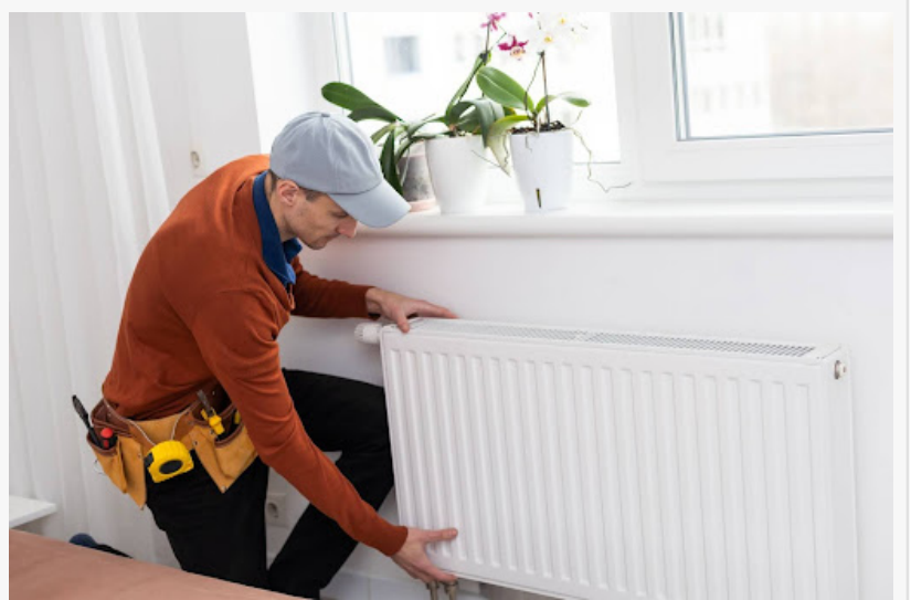
An HVAC technician fitting a radiator to optimize energy savings during professional heating services.
