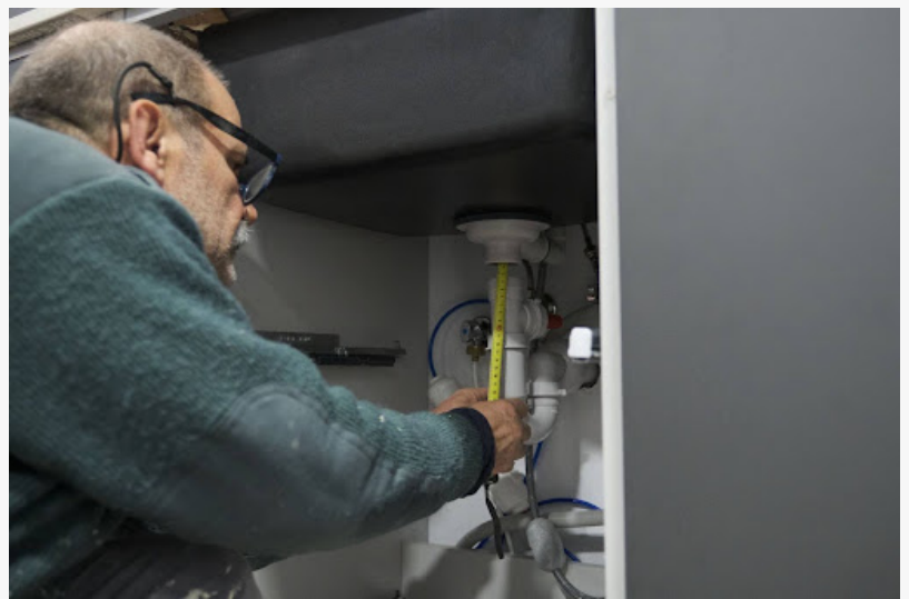
Plumber measuring pipe under kitchen sink to install a sink siphon connected to the garbage disposal unit
