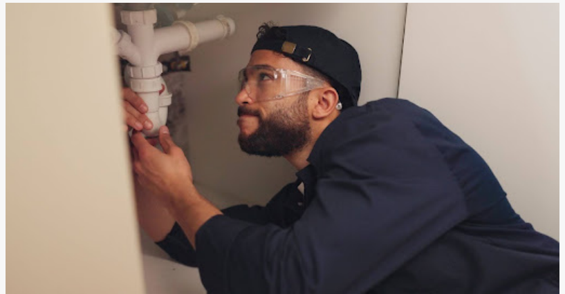
Plumber inspecting kitchen pipes with safety gear before repairing a leak under the sink
