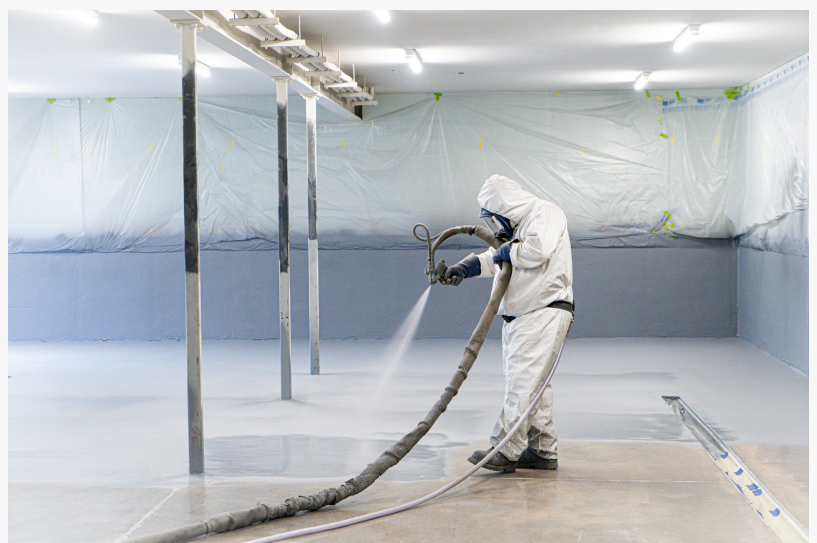
ArmorThane AquaSafe Spray On Application
