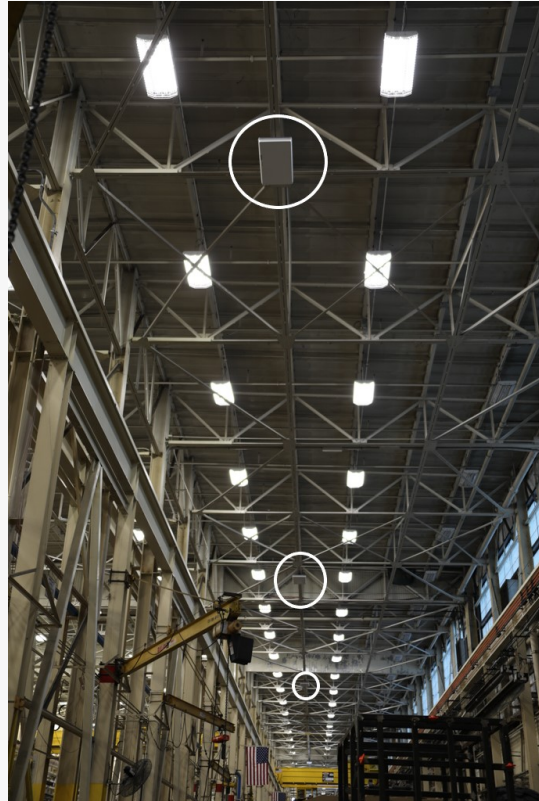
RF Controls' CS-490 RFID-Based RTLS Smart Antennas Installed as Part of MCPIC System
