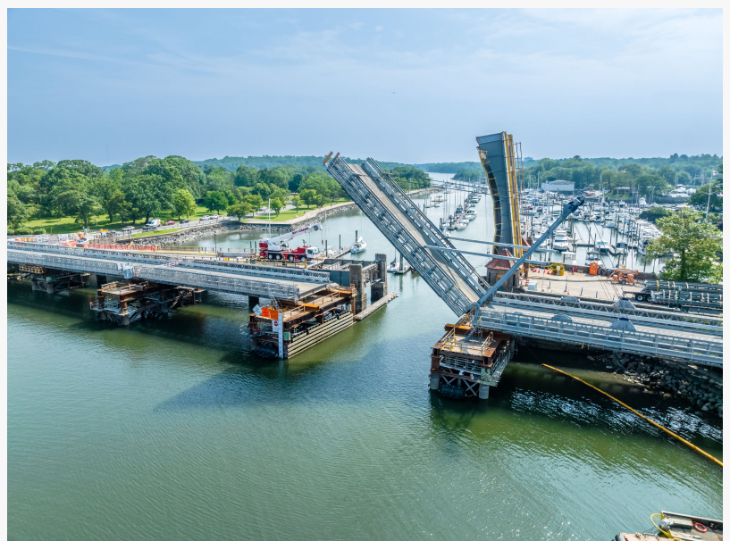
Acrow Temporary Bascule Bridge at Glen Island Park in New Rochelle NY
