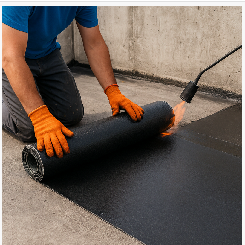
Workers applying advanced waterproofing system to protect concrete surfaces in a Qatar construction project.
