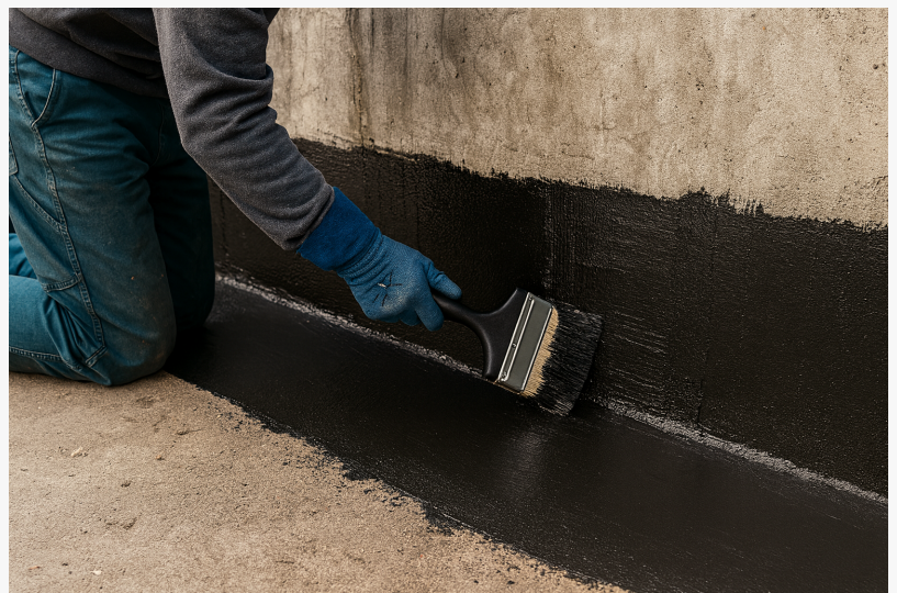
Worker applying a torch-on waterproofing membrane for roof and foundation protection in Doha.
