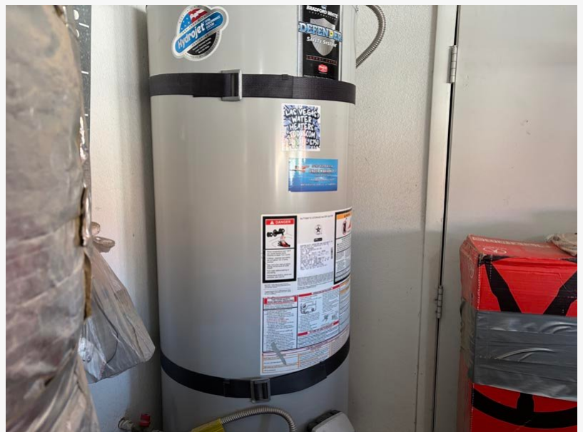
bradford white heater install las vegas valley water heaters today
