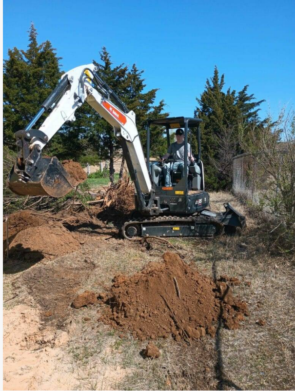
Excavation with Jefferson Land Clearing & Excavation in Jefferson City, TN
