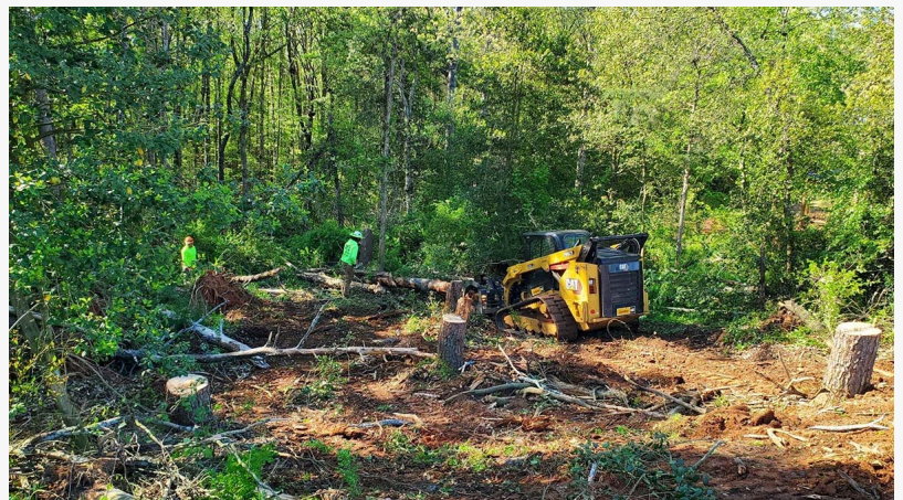
Land Clearing with Jefferson Land Clearing & Excavation in Jefferson City, TN
