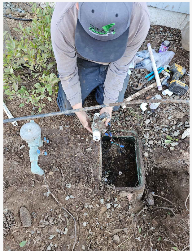
Plumbing Service Job Being Done By Drain Charmer Plumbing & Rooter Inc in Carpinteria
