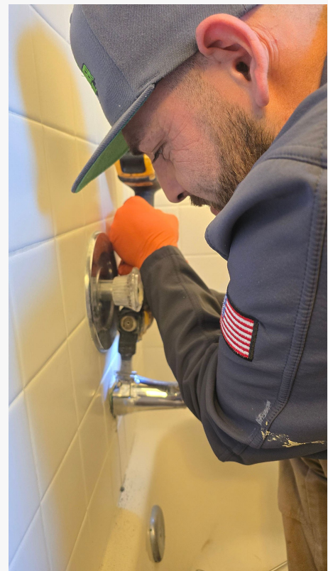
Bathtub and Shower Repair Service Job Done By Drain Charmer Plumbing & Rooter Inc
