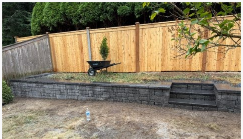
Brand New Landscaping Fence Installed By Ivan's Landscape & Construction
