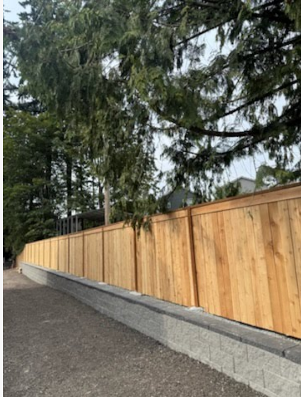
Retaining Wall Installed By Ivan's Landscape & Construction in Snohomish, Washington
