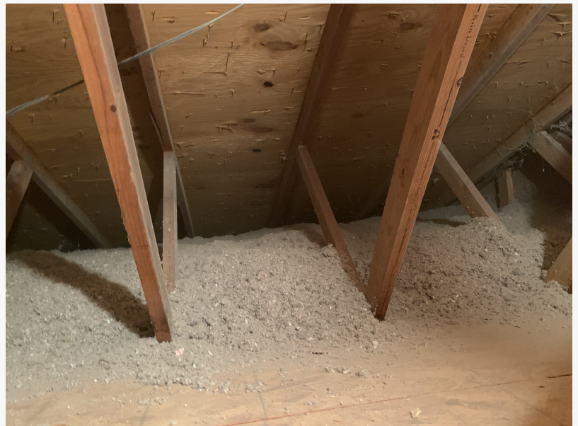
Blown Insulation in an attic
