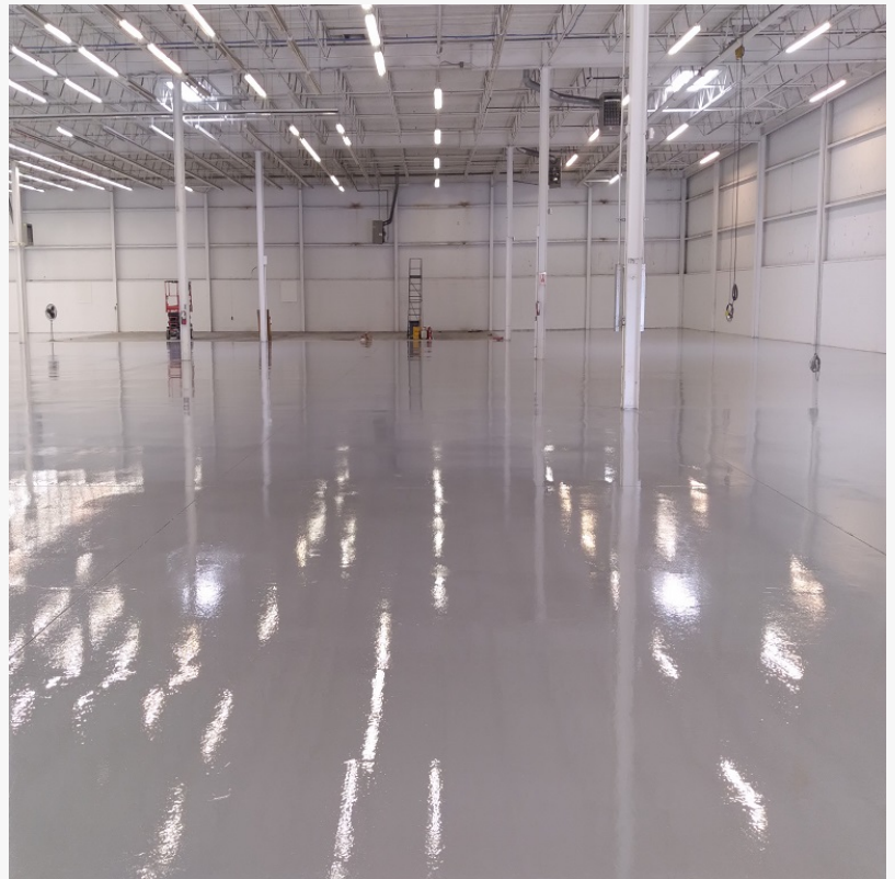
EPOXY FLOORING FOR WAREHOUSE
