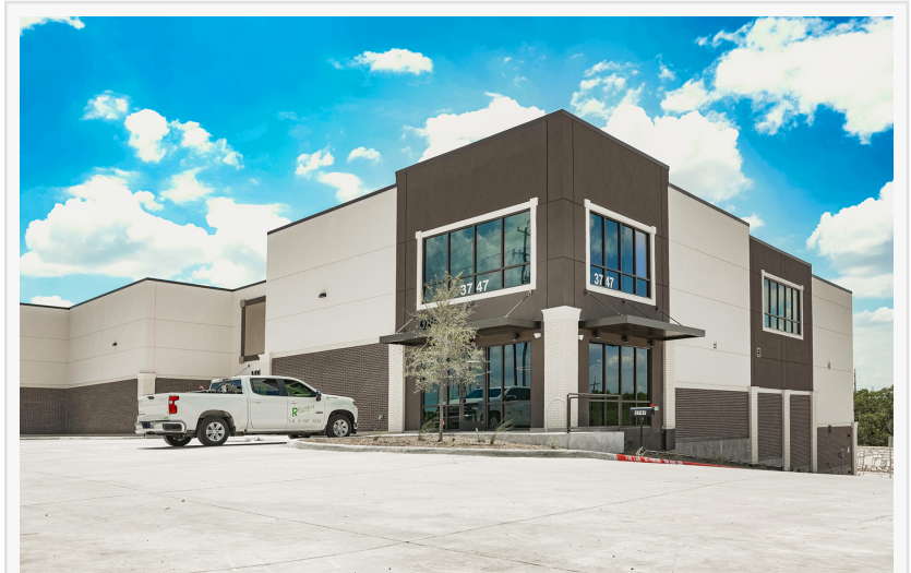
DXD San Antonio has a unique site plan with two levels of ground-floor loading.
