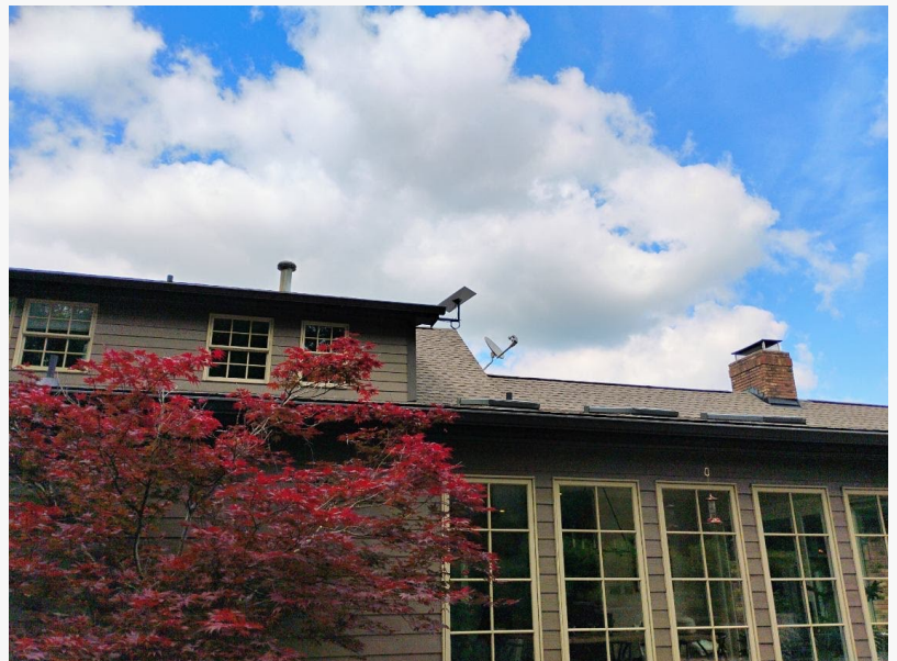
Starlink roof mount set up
