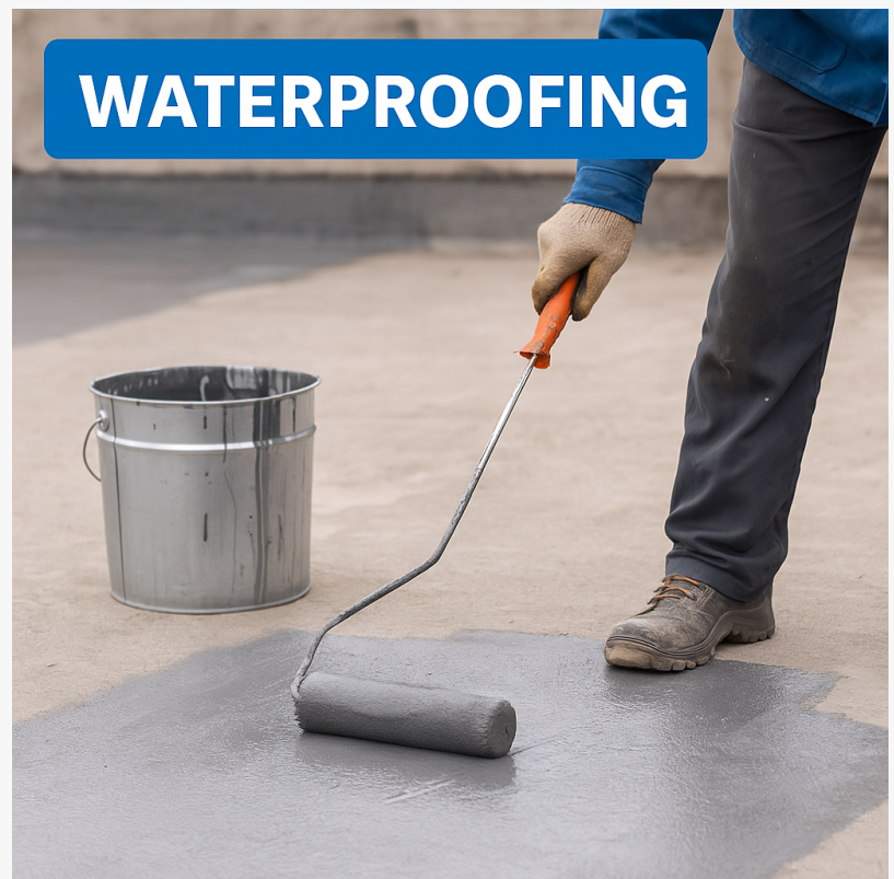
A worker applying liquid waterproofing membrane with a roller on a commercial building roof.
