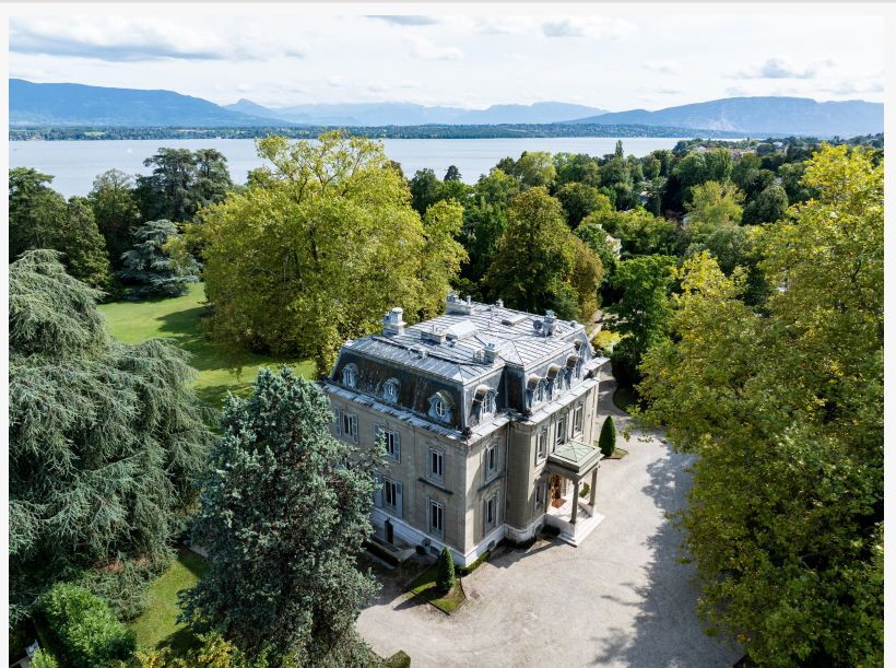
Historic 1867 Second Empire Mansion by Architect Francis Gindroz
