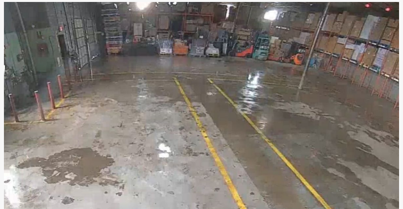
Before Warehouse Resin Flooring
