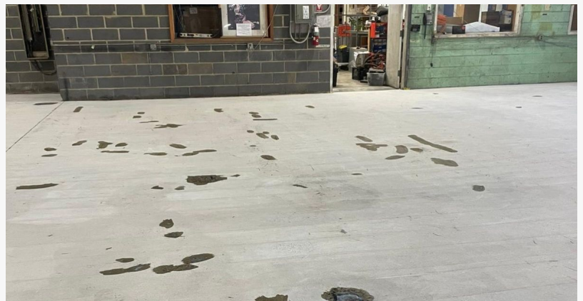
During Warehouse Resin Flooring
