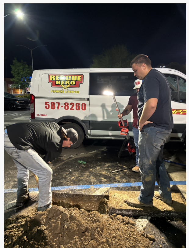
Rescue Hero Plumbing team digging to install a new sewer line in Bakersfield, CA.
