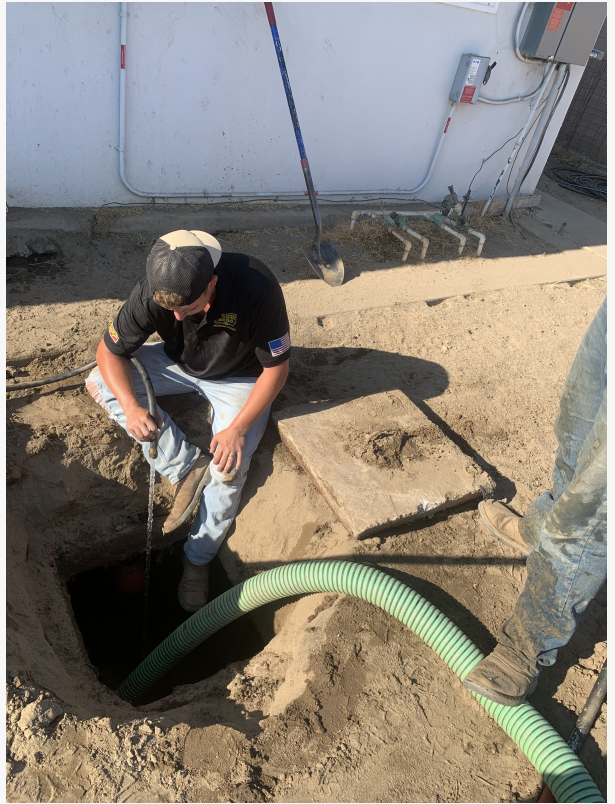
Rescue Hero Plumbing crew watering a hole during septic system preparation in Bakersfield, CA.
