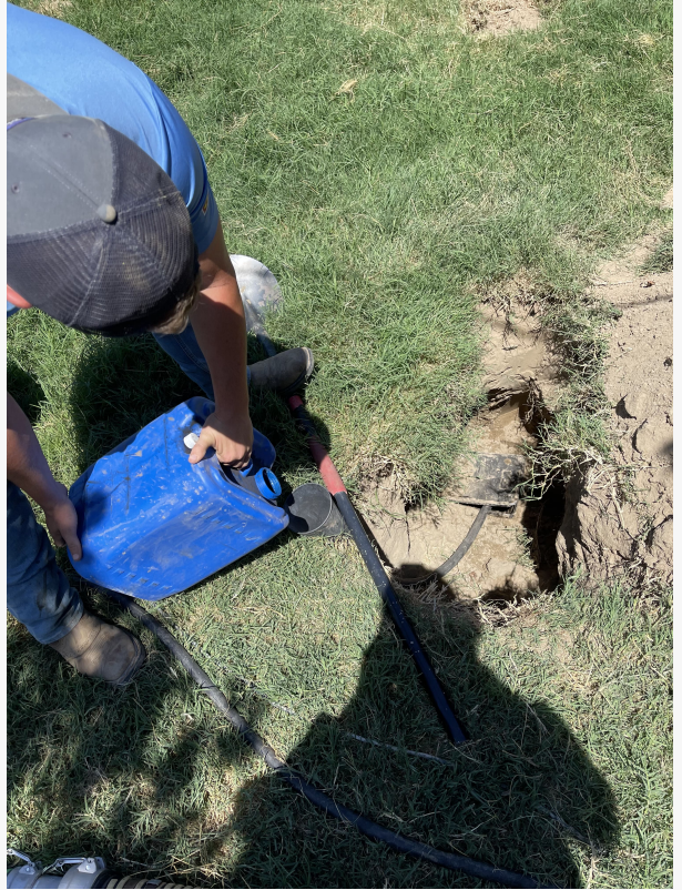
Rescue Hero Plumbing crew prepping a site for septic system work in Bakersfield, CA.
