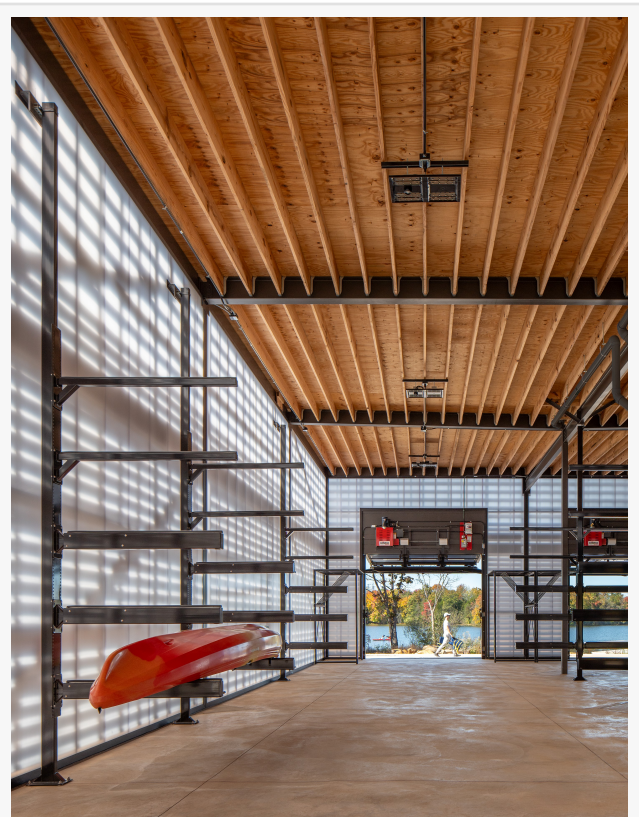
Six local high school rowing teams utilize the new boathouse. The polycarbonate exterior provides aesthetics, safety, and energy efficiency. Photo: Allen Russ Photography, LLC, Studio HDP copyright.
