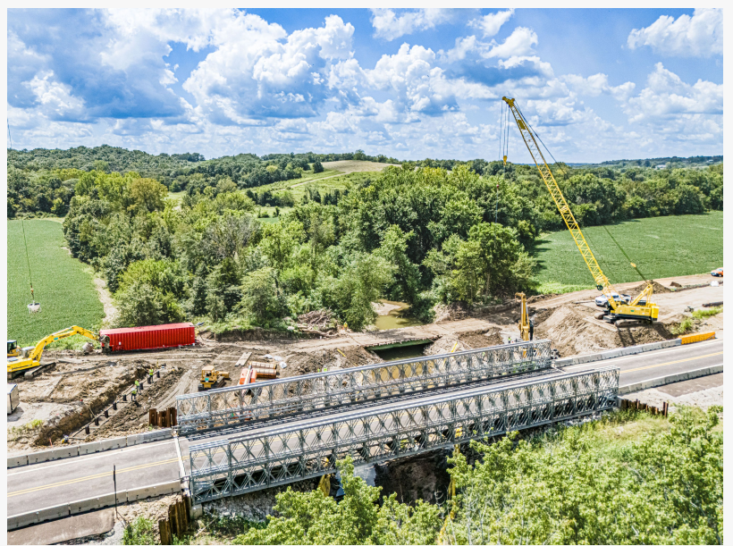
Acrow Bridge in service in Southern Iowa
