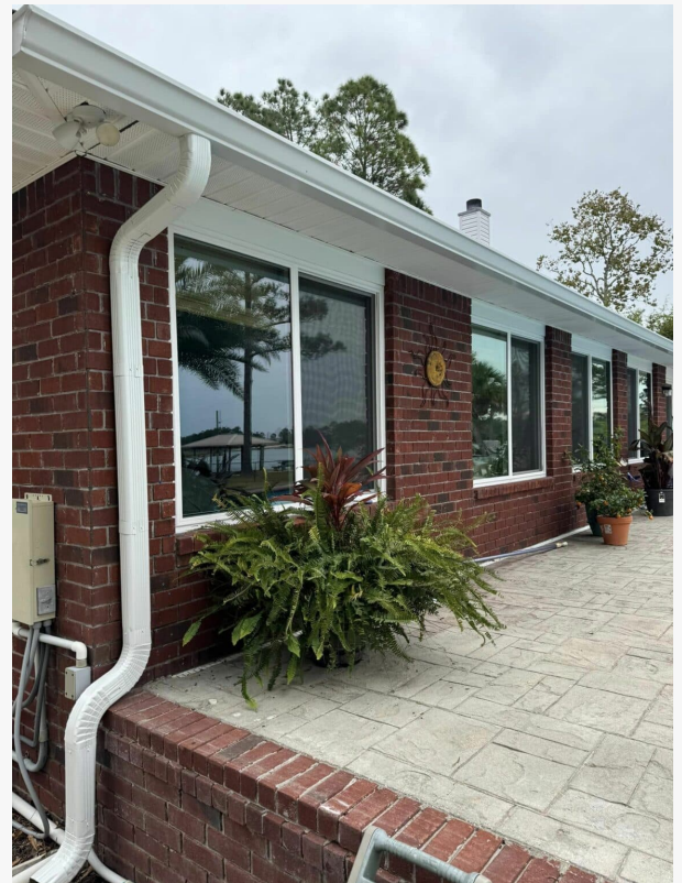
Gutter Installation Pensacola
