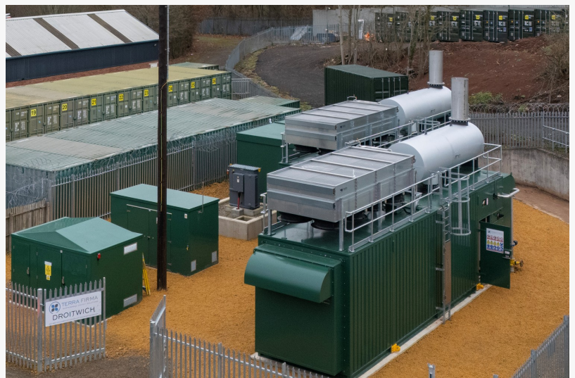
Terra Firma Energy's Droitwich Spa plant generates electricity to the grid with 2 MTU Hydrogen ready gen sets
