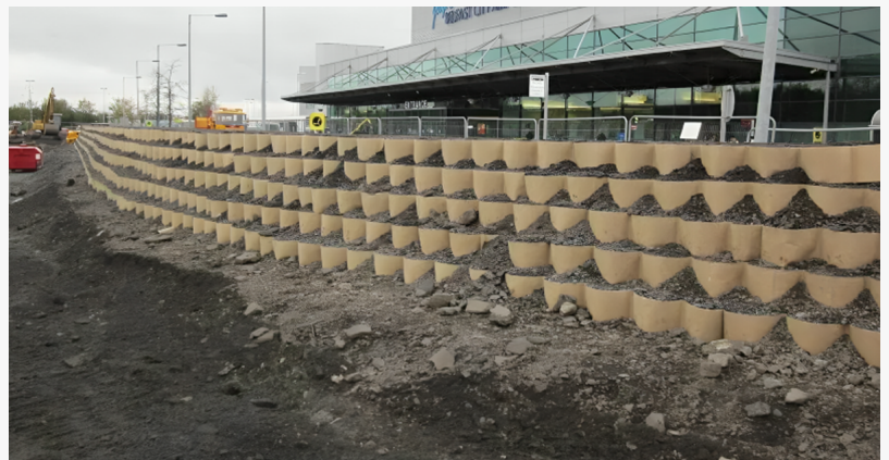
flood proof walls
