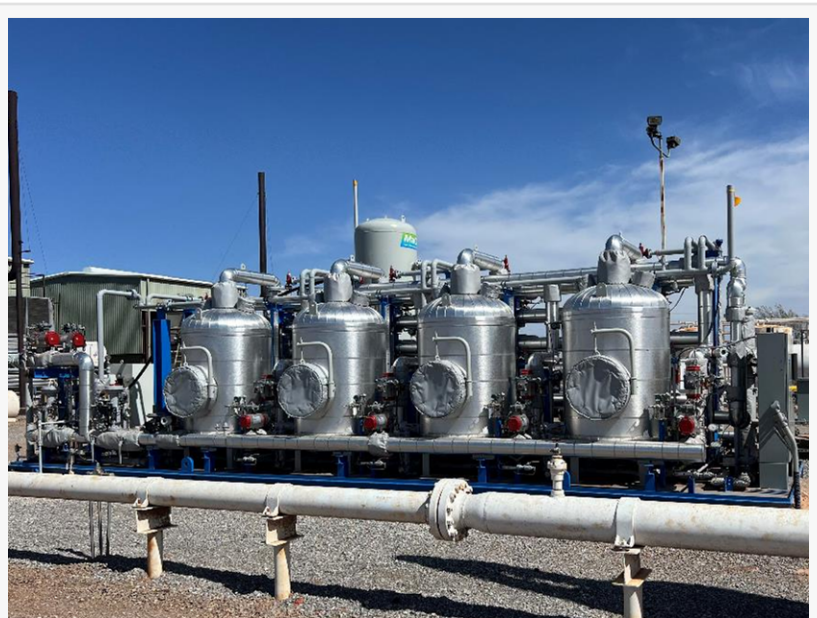
ColdStream Energy's MaCH4 NGL Recovery Solution, a key technology in natural gas processing, designed to capture and recover valuable natural gas liquids (NGLs) while minimizing emissions and maximizing efficiency
