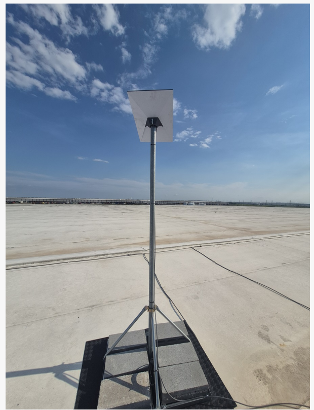
Starlink Installation for Business by ProSat Networks 1-844-799-0258
