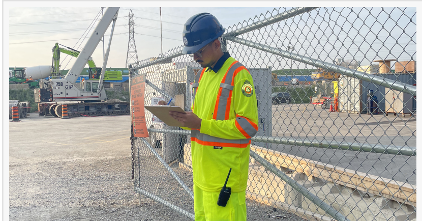
G Force commercial security guard making reports at the constructions site
