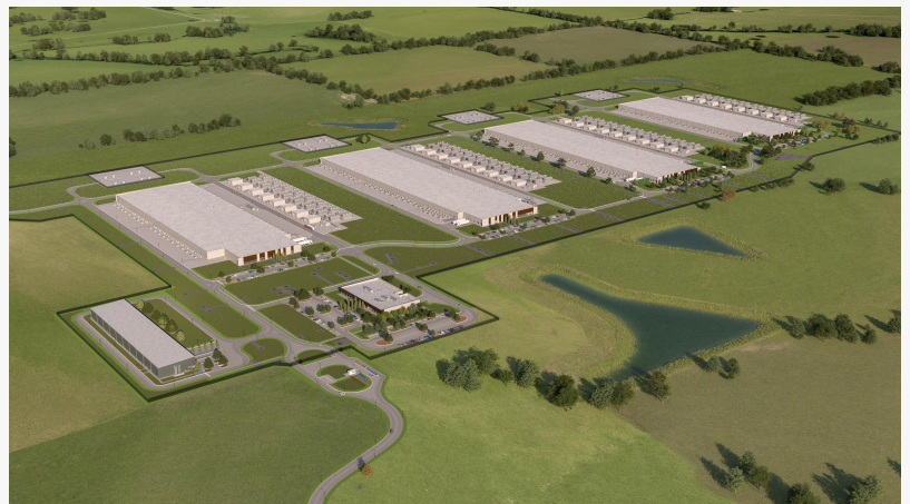
Rendering of Meta's expanded data center campus in Montgomery, part of the company's $1.5 billion investment in Alabama's Capital Region.
