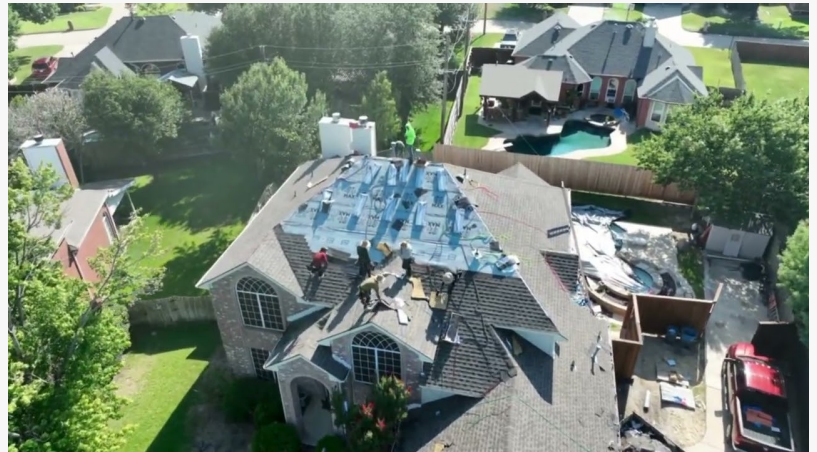
Roofing crew installing new shingles and protective underlayment on a large residential home during a full roof replacement project.
