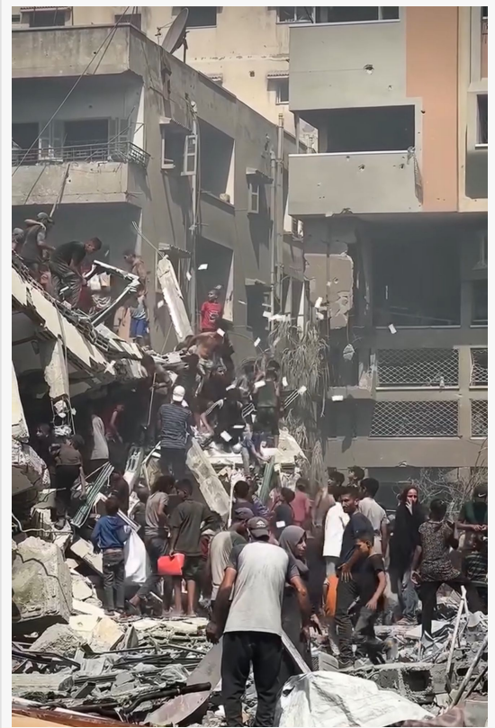
Destruction by Israeli Forces of Al Shawa building out of which medical relief offices and charities were functioning.
