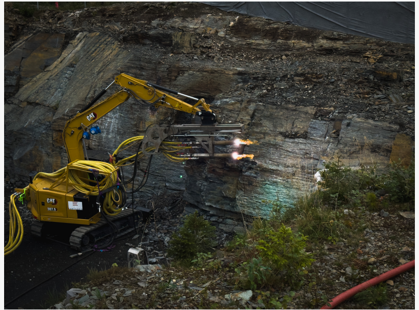
EarthGrid's Plasma Excavation System (PES) in action, in Norway.
