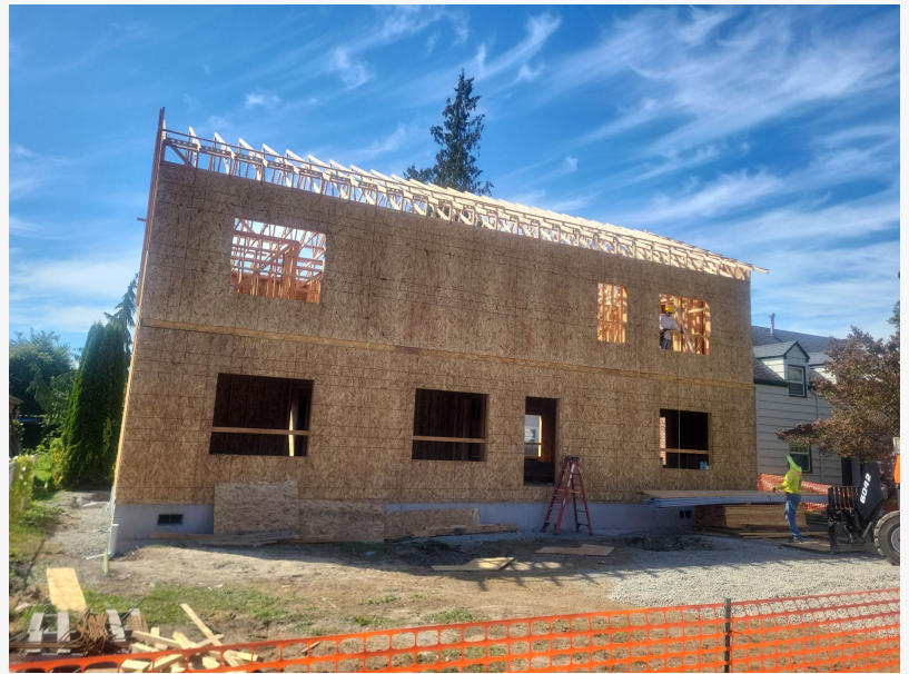
Chad Fisher Construction of New Earth Recovery Cedar House #2
