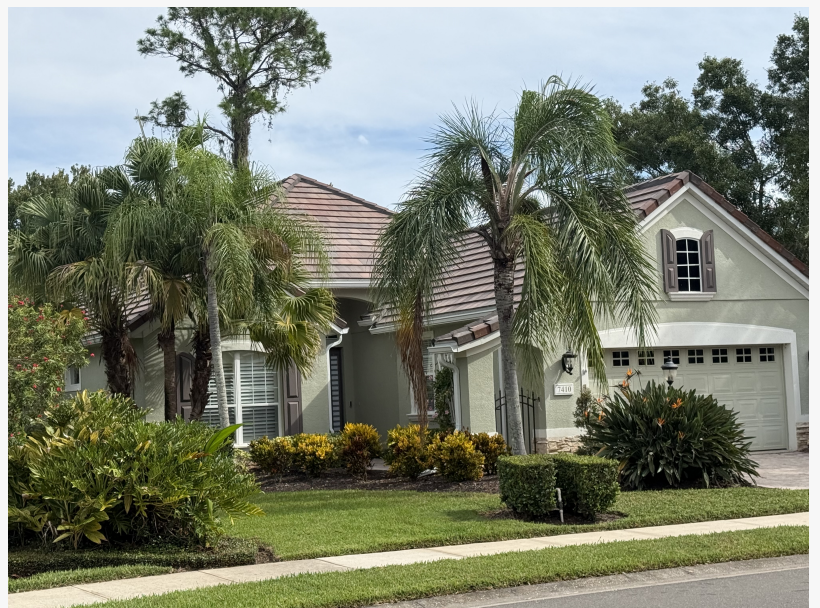
A recently completed FORTIFIED™ Roof installed by Beardman Building Services in Bradenton, FL
