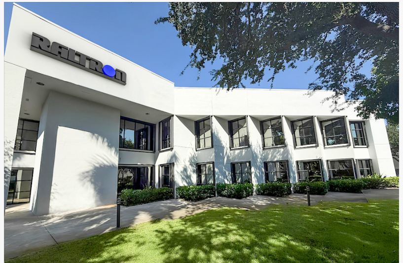
New Raltron Production Facility in Miami
