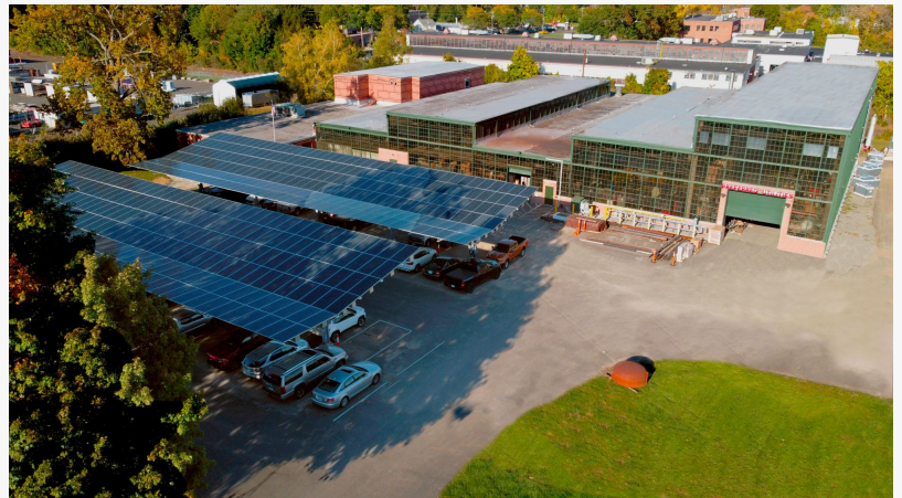
Preferred Utilities' Danbury, Connecticut headquarters
