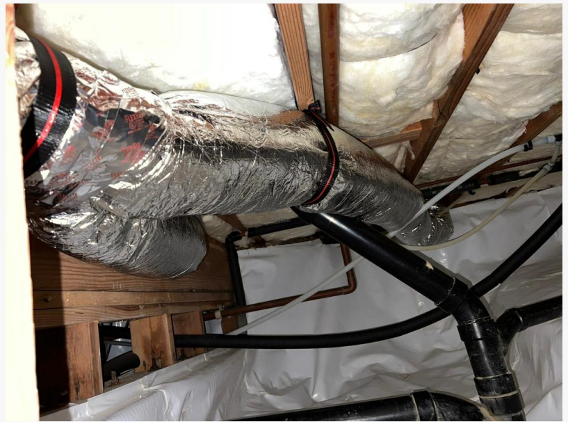
Crawl Space Encapsulation Los Angeles
