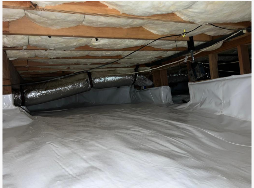
Crawl Space Vapor Barrier
